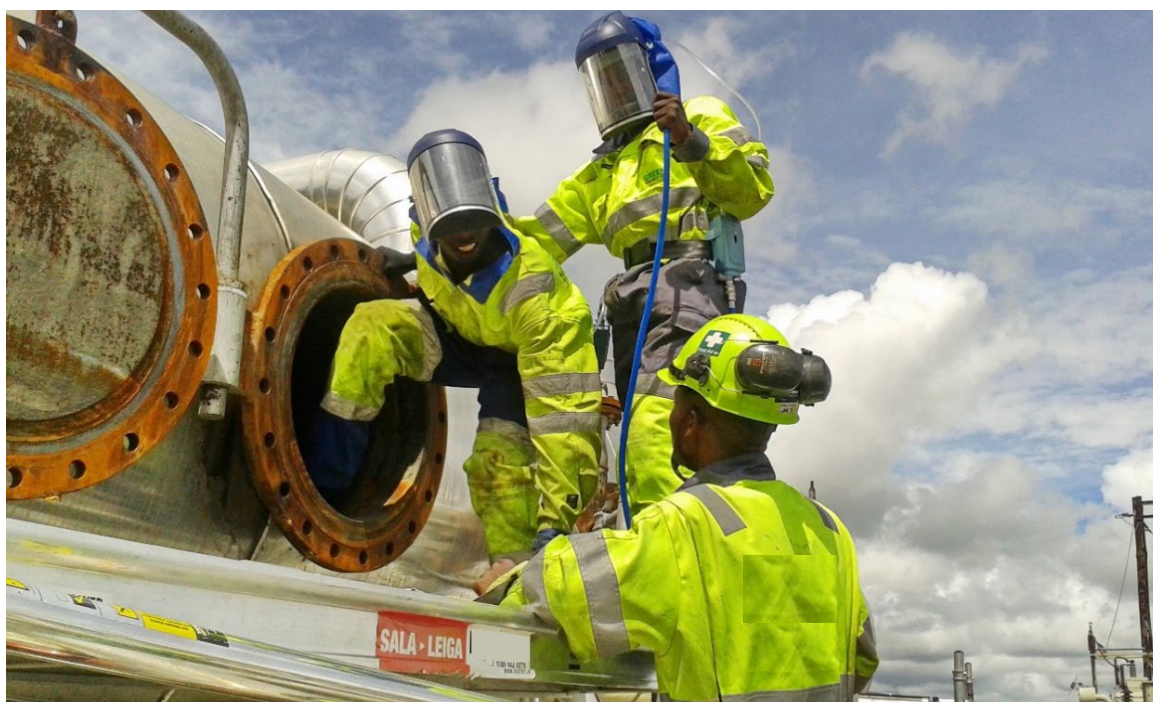
Photo: Welders working on a geothermal project in Kenya
