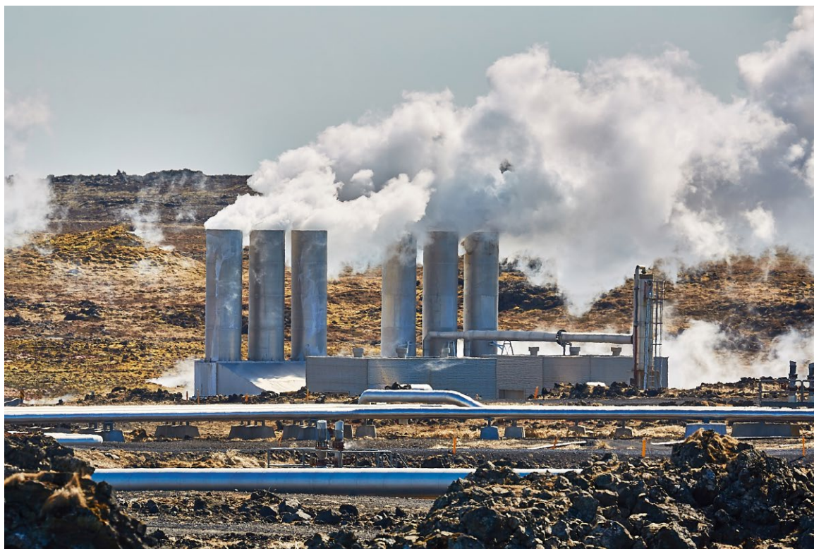
Photo: Geothermal power plant
